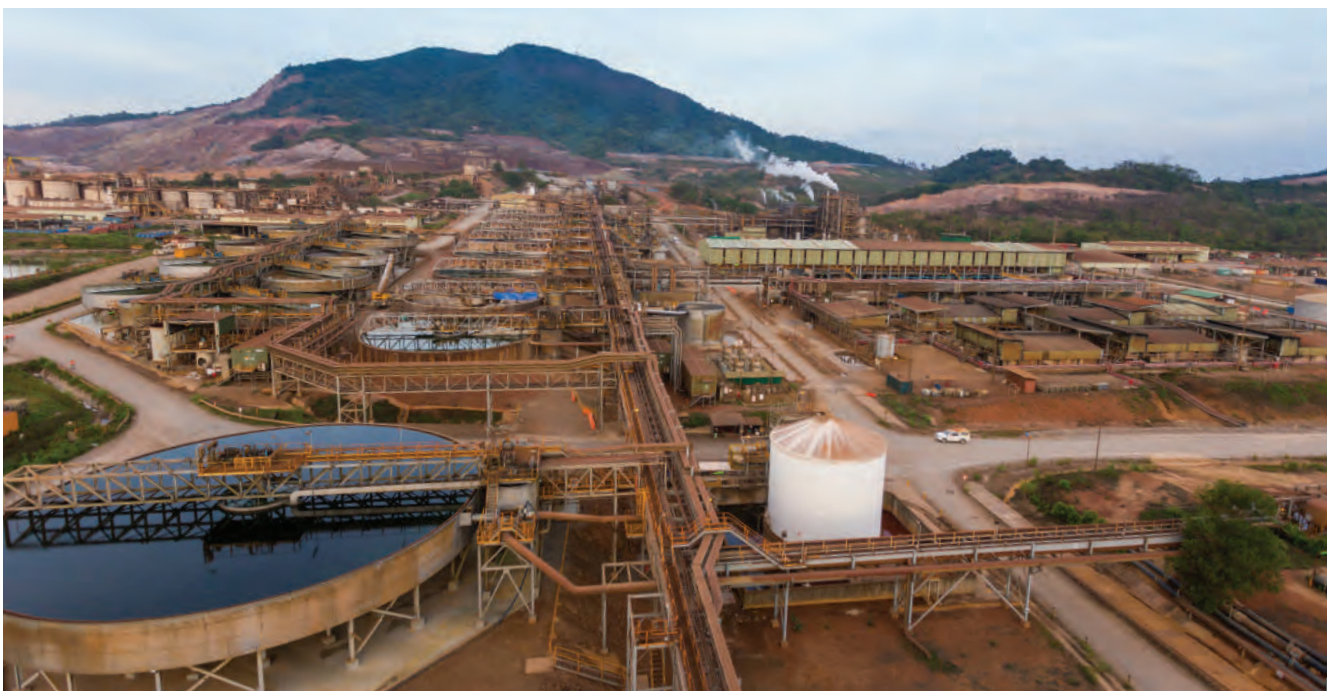
IMAGE: Processing facility at Sepon.
