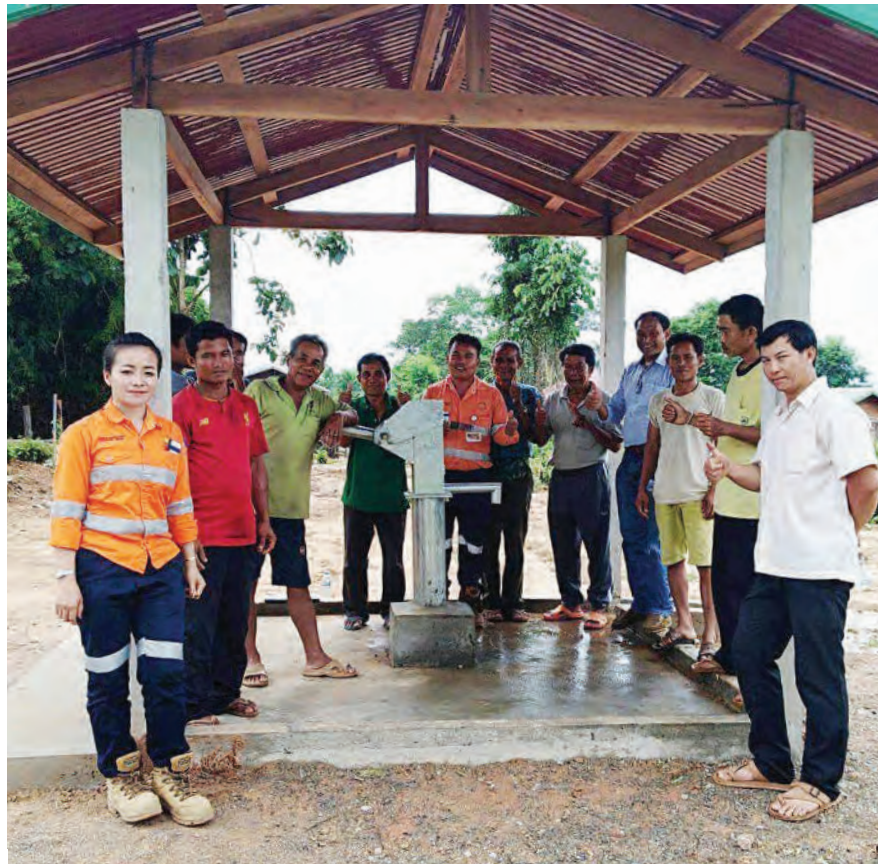
IMAGE: Potable water infrastructure in a community near Sepon.
