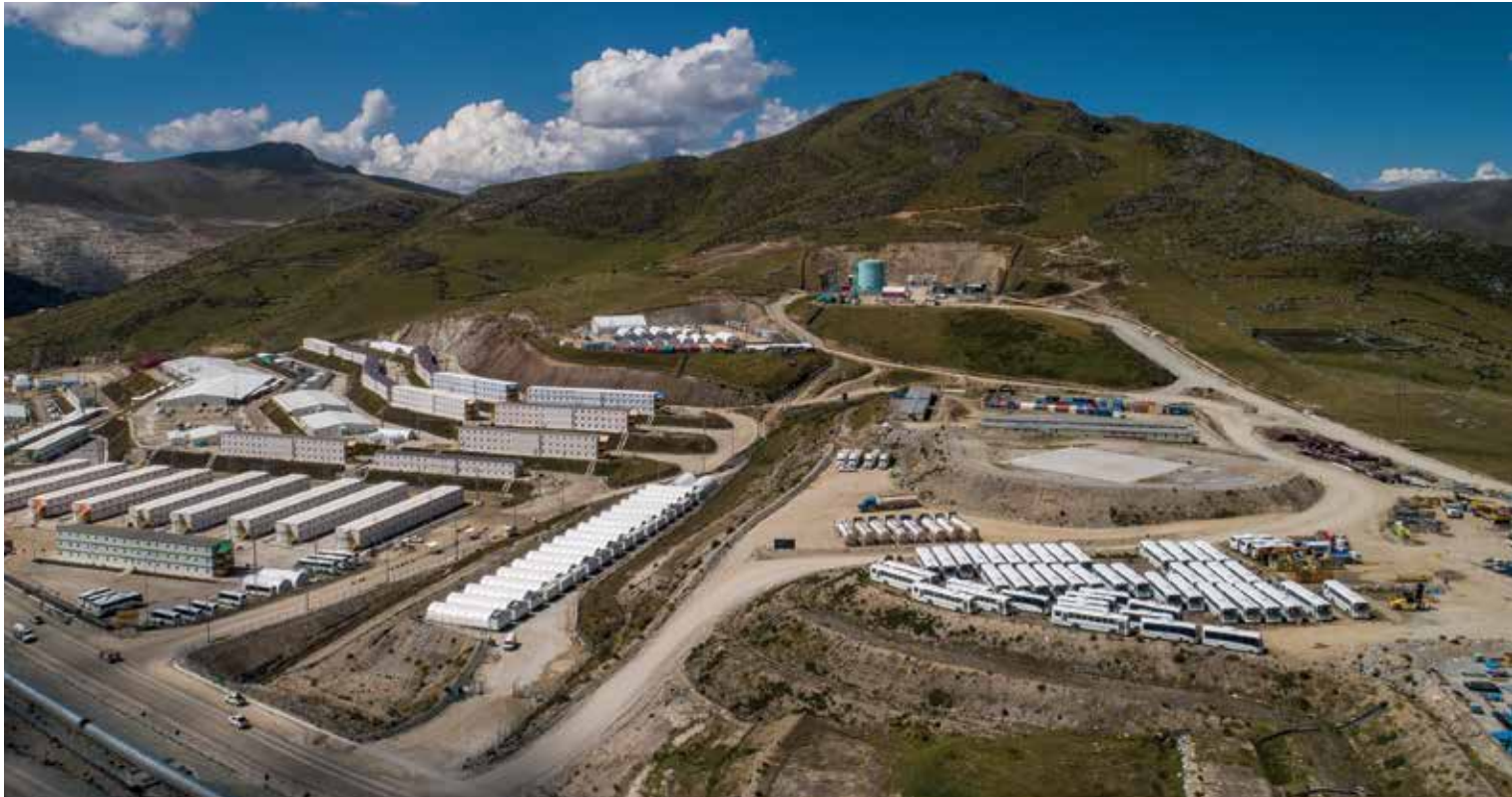
Located at 4,000 metres above sea level, the Anta Wasi Camp houses our employees.
