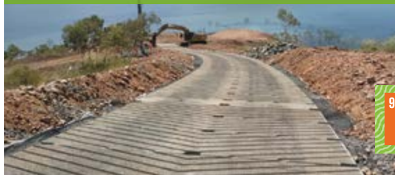
IMAGE: TSF access road, Dugald River, Australia.
