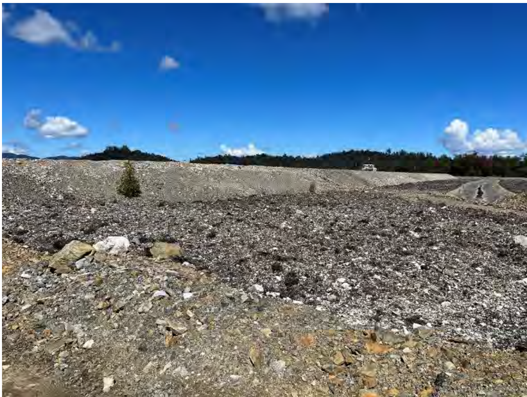
Photograph 12 – Trial cover area, north wall (RL 199 m), looking west.
