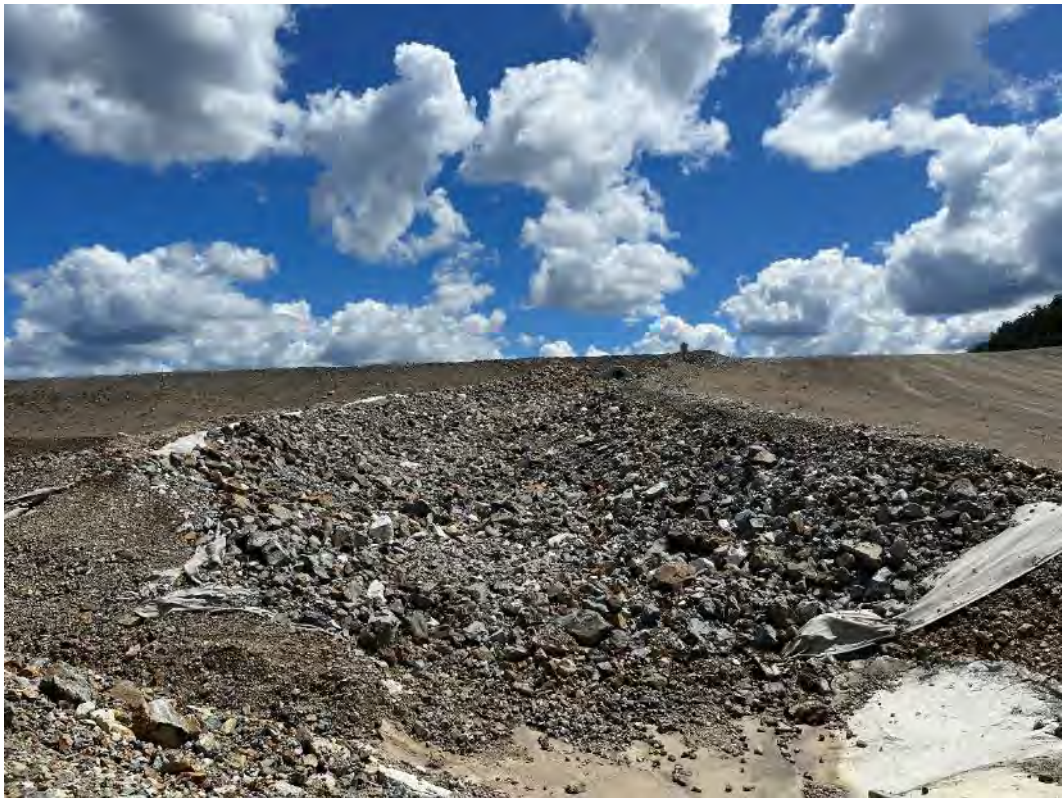
Photograph 2 – Southern access ramp
