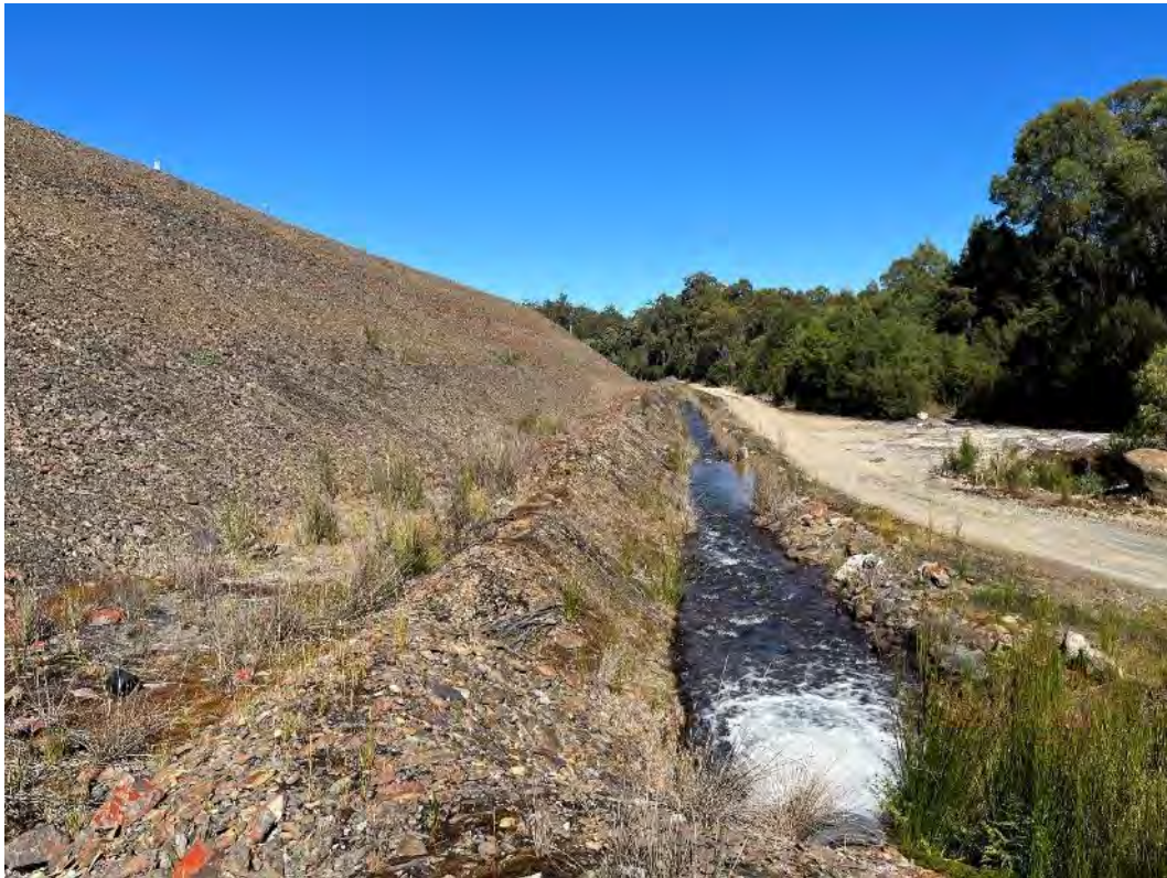
Photograph 9 – Decant channel, looking west from outlet pipe.
