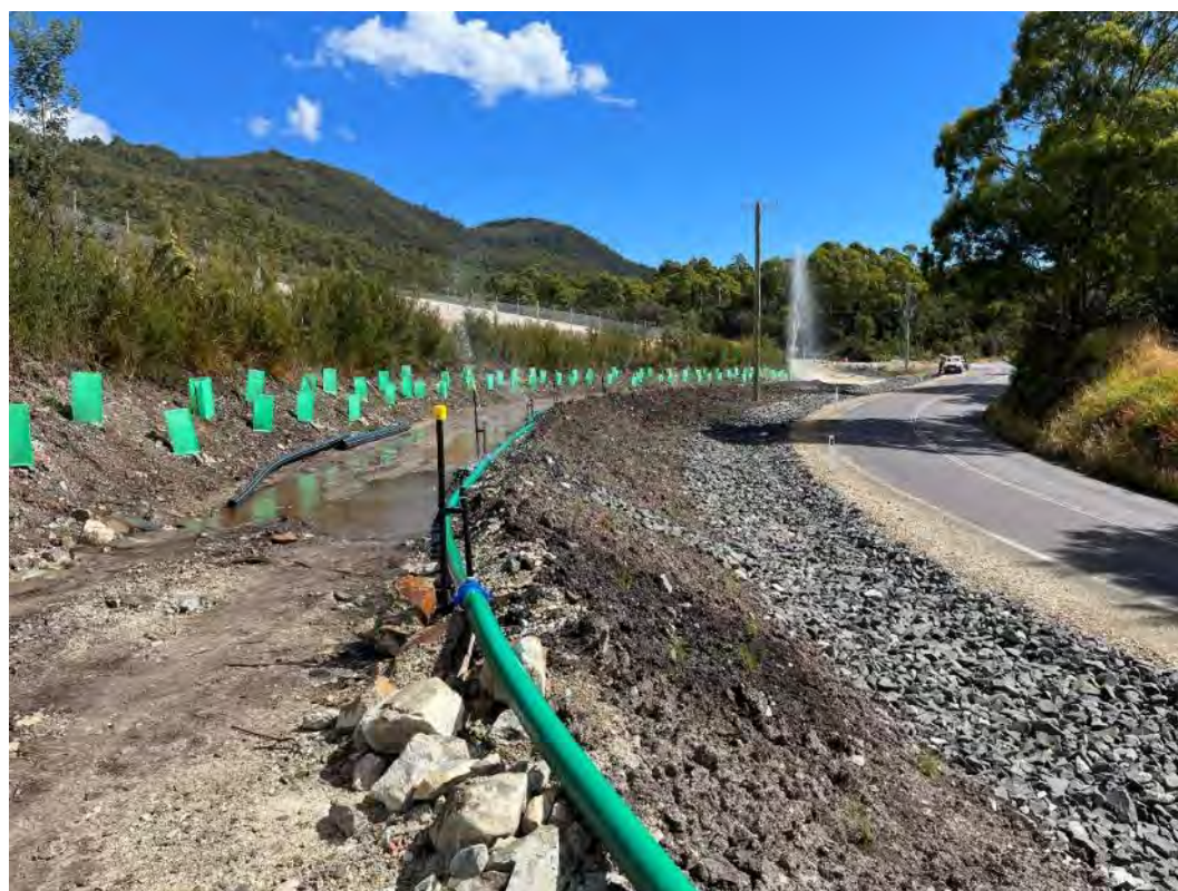
Photograph 34 –downstream area of screening bund, adjacent to Murchison Highway.
