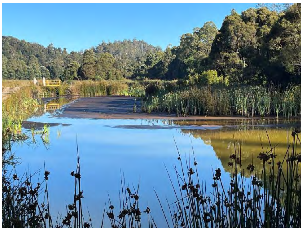
Photograph 40 – Polishing Pond Cell 3. Large amounts of sludge have accumulated within several cells.
