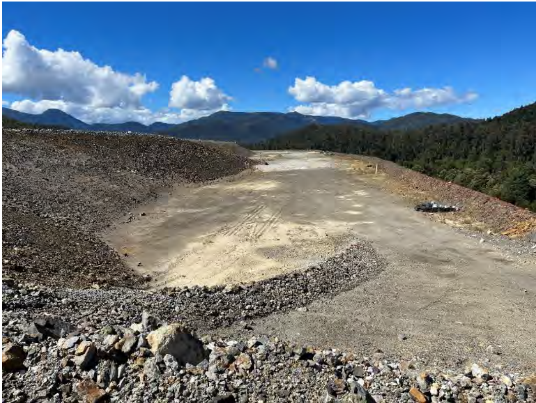
Photograph 31 –western buttress overview, note wind blown tailings.
