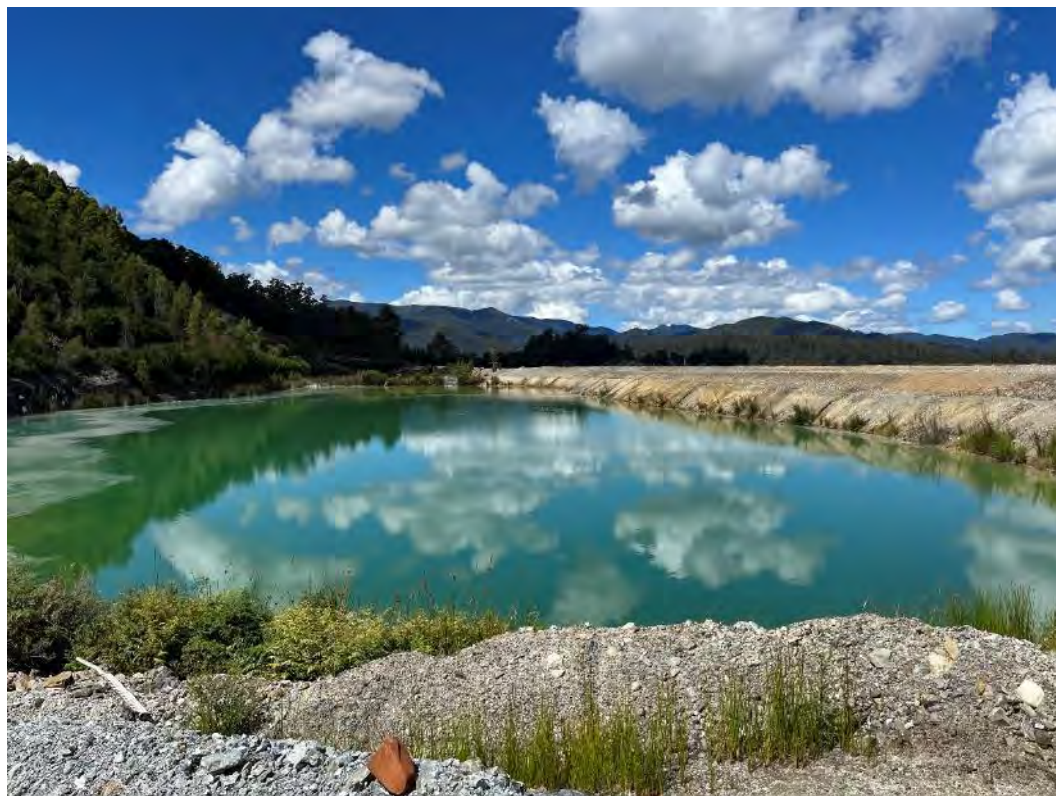
Photograph 17 – Overview of decant pond, looking south.
