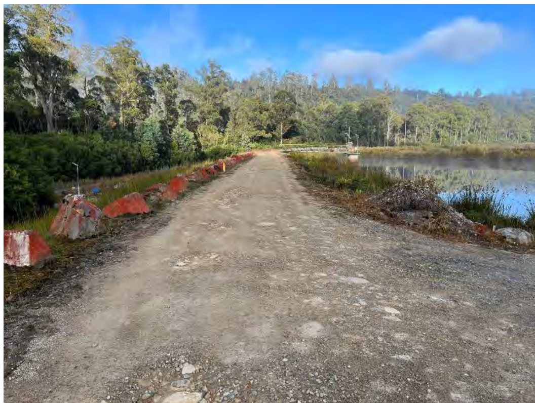
Photograph 36 – Polishing Pond – typical condition of the crest
