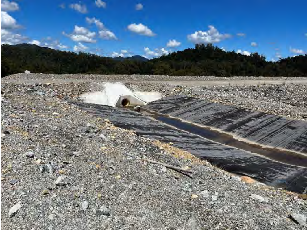
Photograph 21 – Western soil cover outlet drain and culvert.
