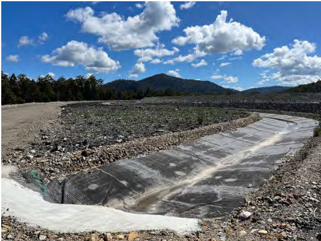
Photograph 20 - Western soil cover outlet drain.
