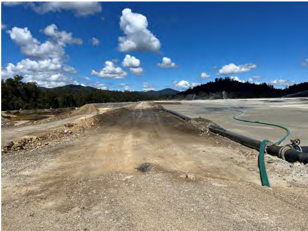
Photograph 22 – Crest of southern embankment (Stage 10), looking west.
