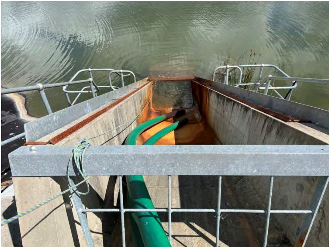
Photograph 25 – decant, clear of obstructions
