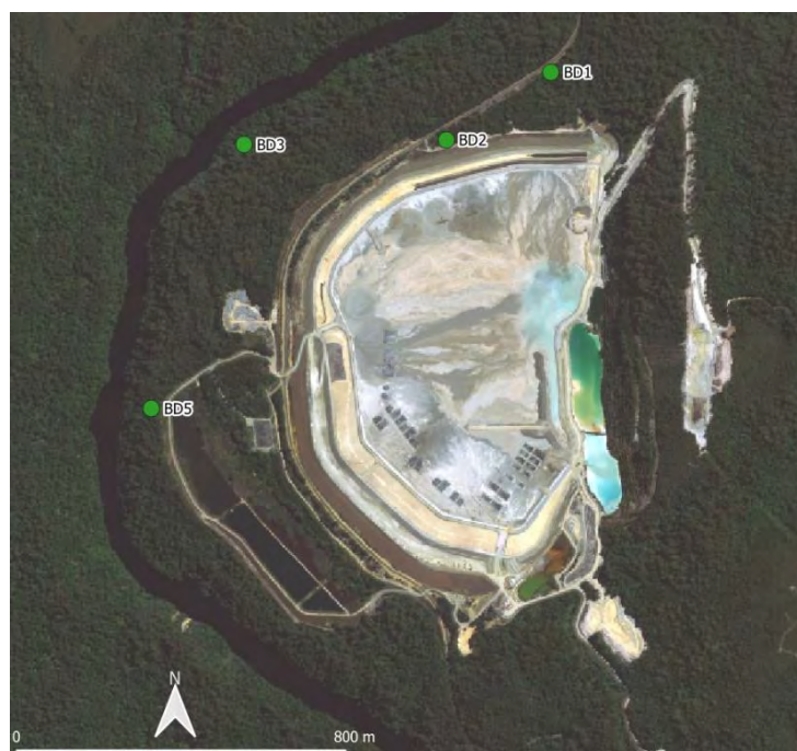
Figure 5-1. Seepage monitoring locations at Bobadil TSF.
