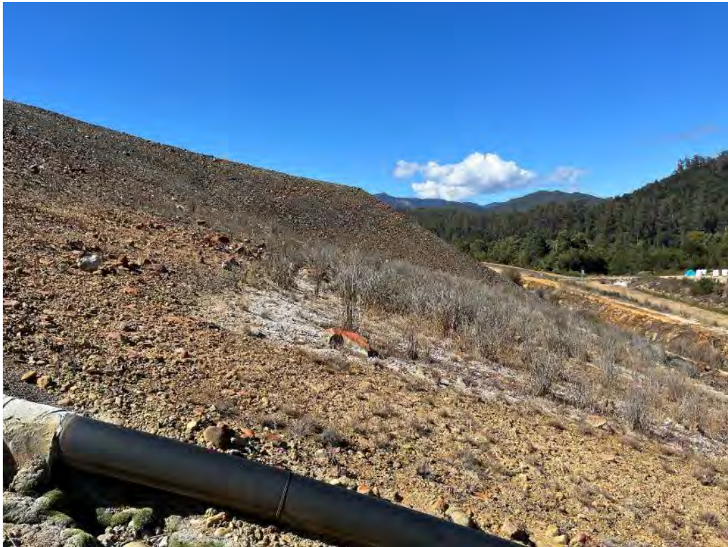
Photograph 29 – reeds on downstream batter of Levee embankment signify the upper extent of broad wet area.
