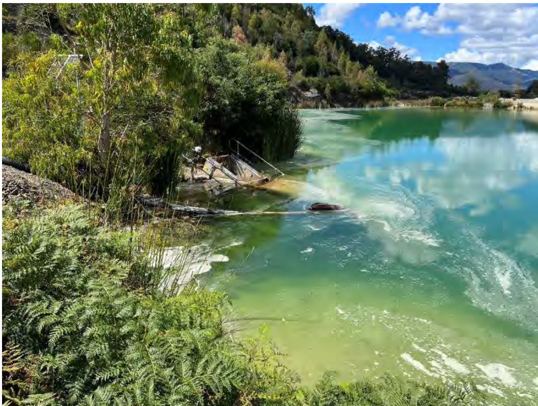
Photograph 16 – Overview of decant, clear water being decanted.
