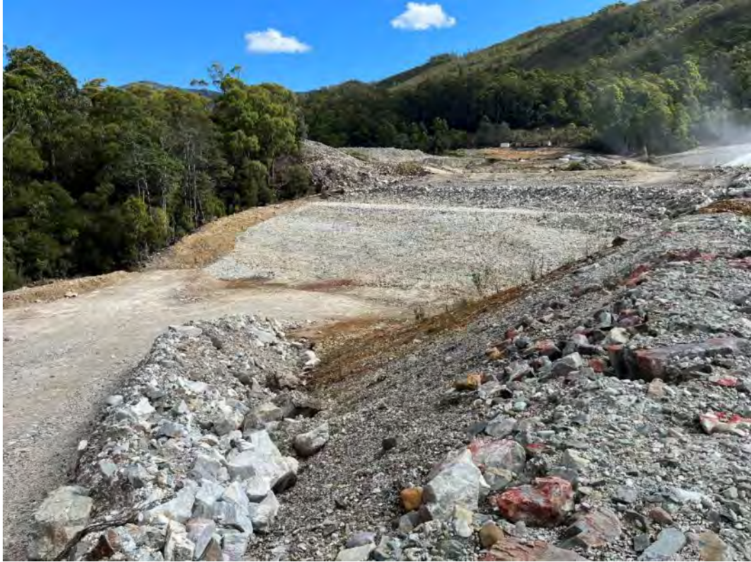
Photograph 7 – filter bund downstream of eastern embankment within old CWDD.
