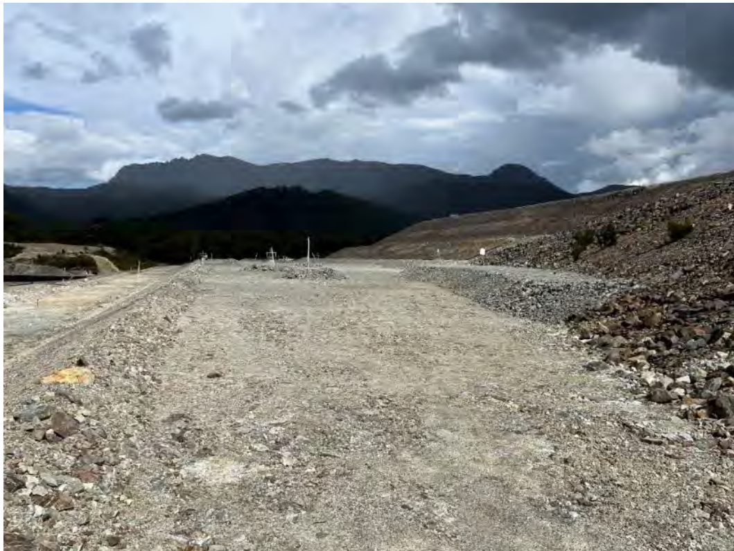
Photograph 21 – northern embankment lower bench.
