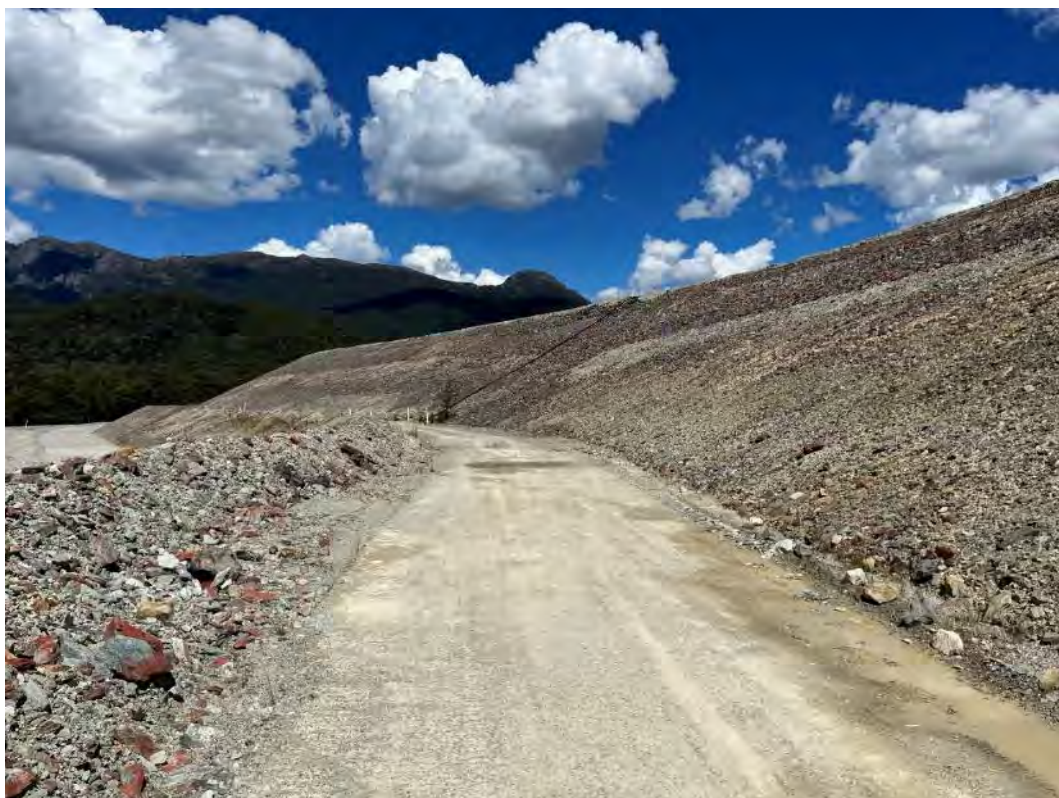
Photograph 22 – downstream slope of northern embankment looking east, good condition.
