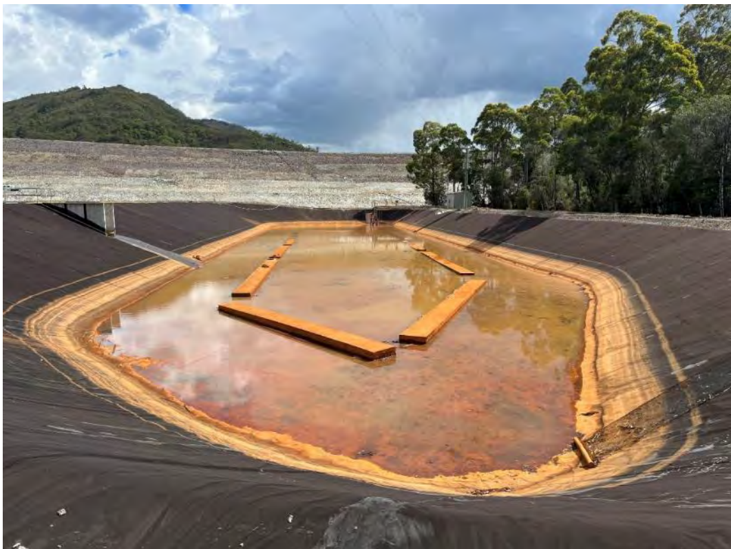
Photograph 16 – overview of lower SCP, looking south from north.
