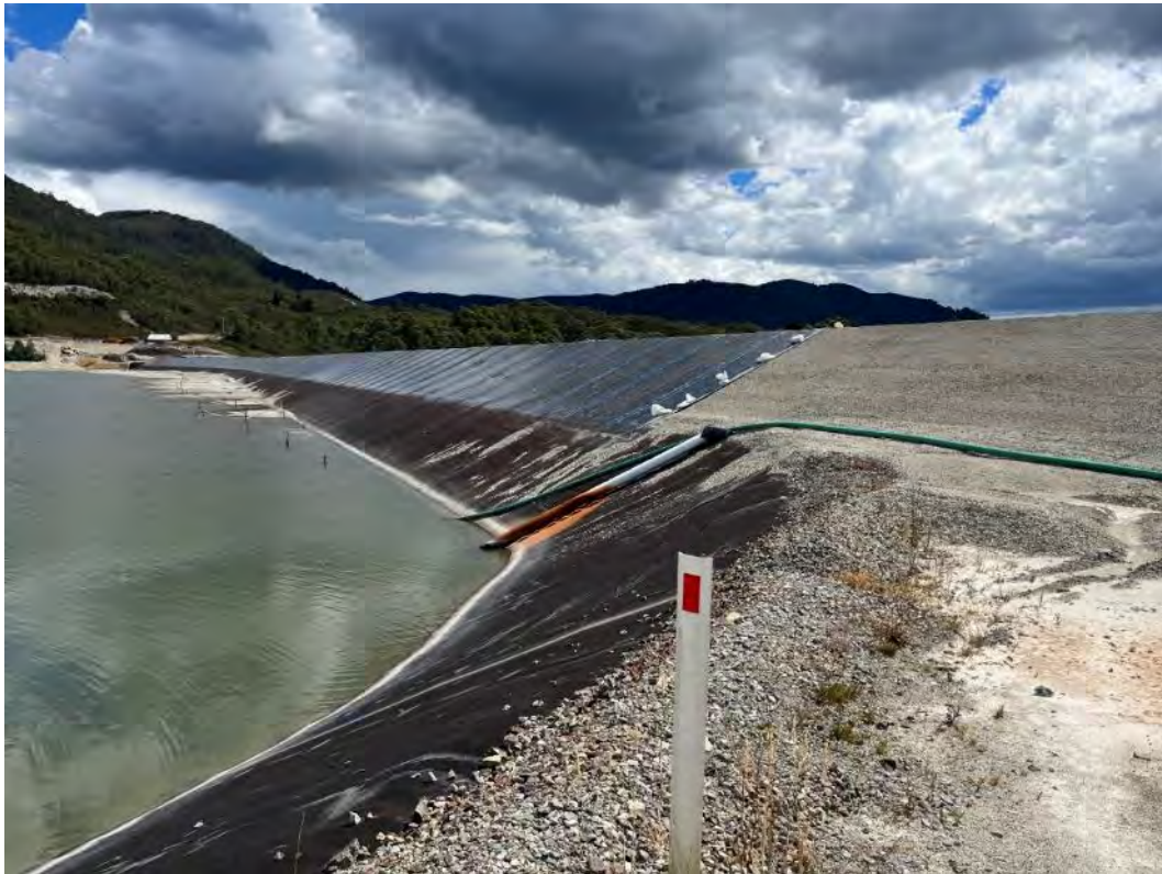
Photograph 23 – upstream face of western embankment, looking south. Stage 2 raise recently completed.
