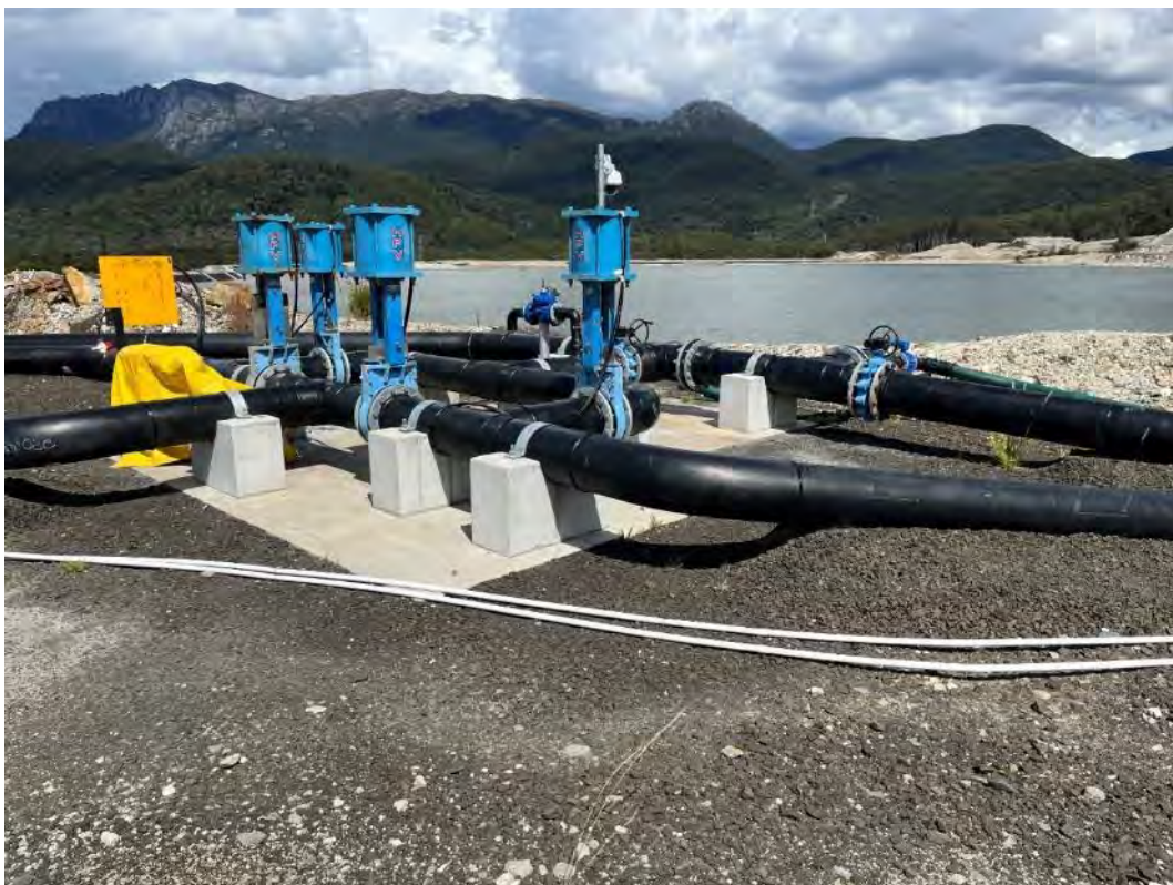
Photograph 28 – Footing at valve station has been repaired since previous inspection.
