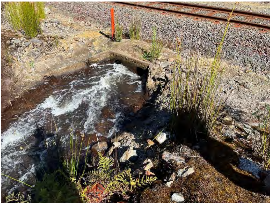
Photograph 8 – bypass drain culverts beneath rail.
