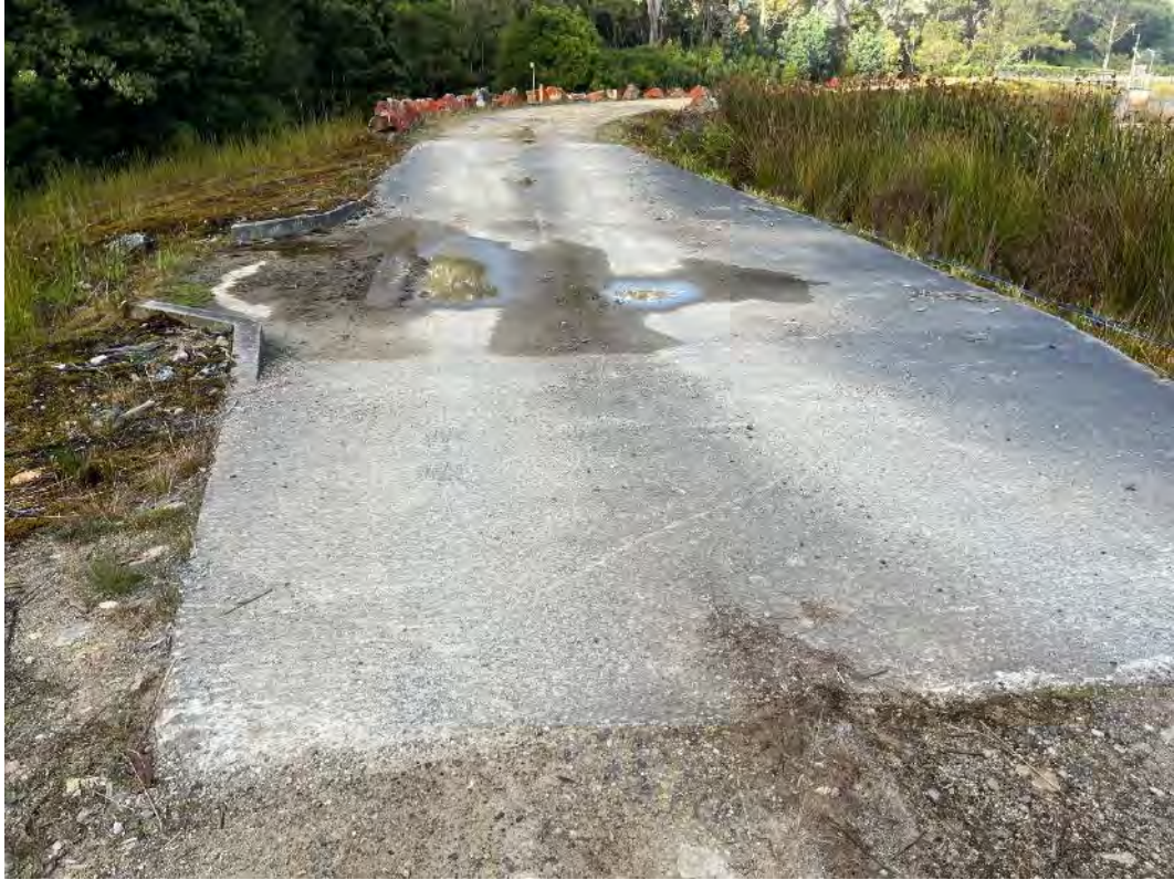
Photograph 41 – Polishing Pond embankment concrete spillway.
