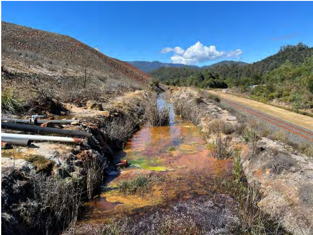
Photograph 15 – condition of the old decant drain, looking south from headwall.
