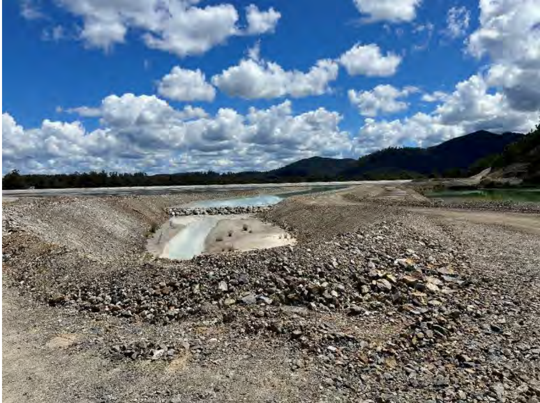
Photograph 19 – New Decant approach channel showing energy dissipation weir.
