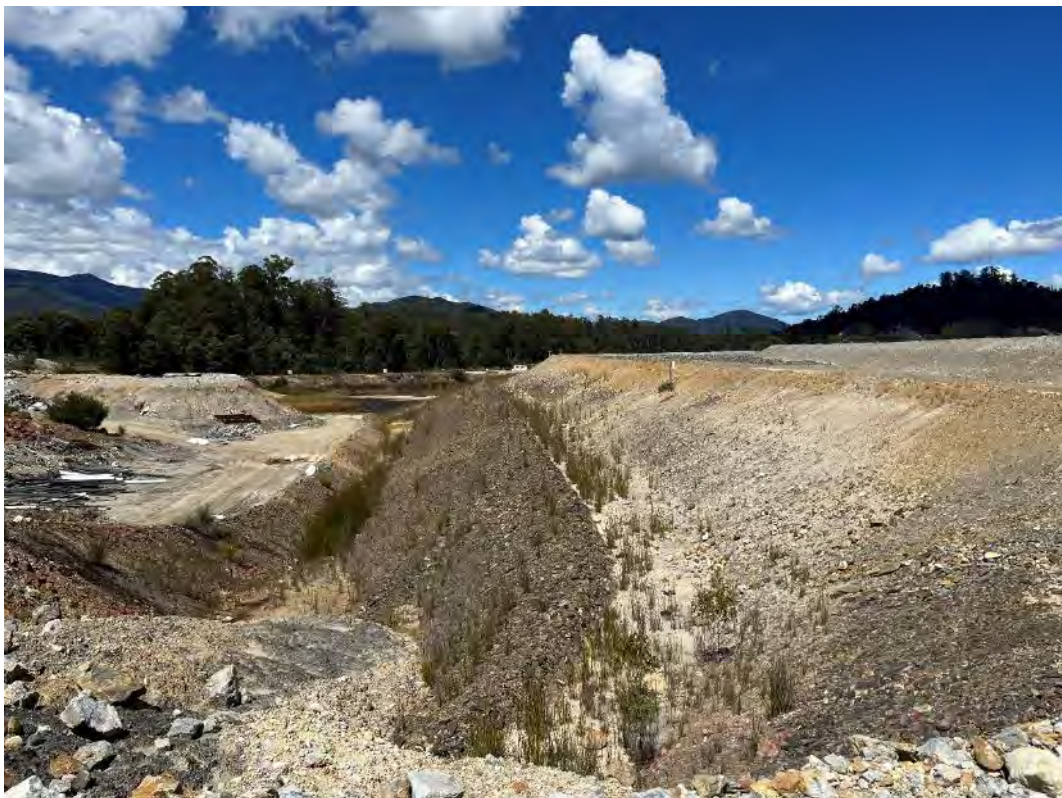
Photograph 4 – Southern embankment downstream slope
