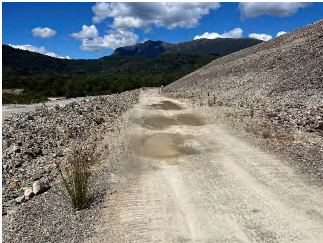
Photograph 20 – northern embankment bench, pooling water, looking east.
