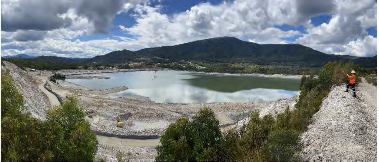
Photograph 37 – overview of 2/5 Dam from CWDD.
