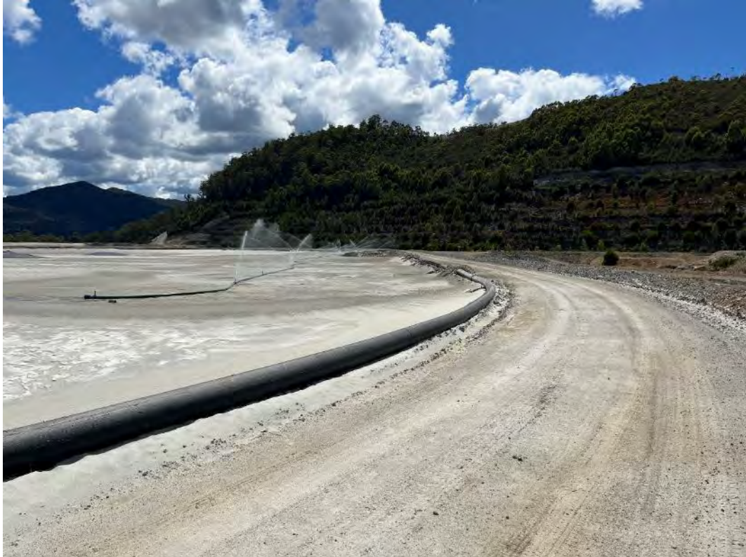
Photograph 5 – overview of downstream slope of northern embankment, looking south
