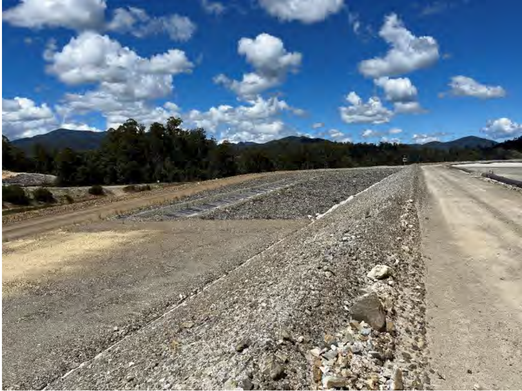
Photograph 1 – Southern embankment downstream slope and soil cover ara.
