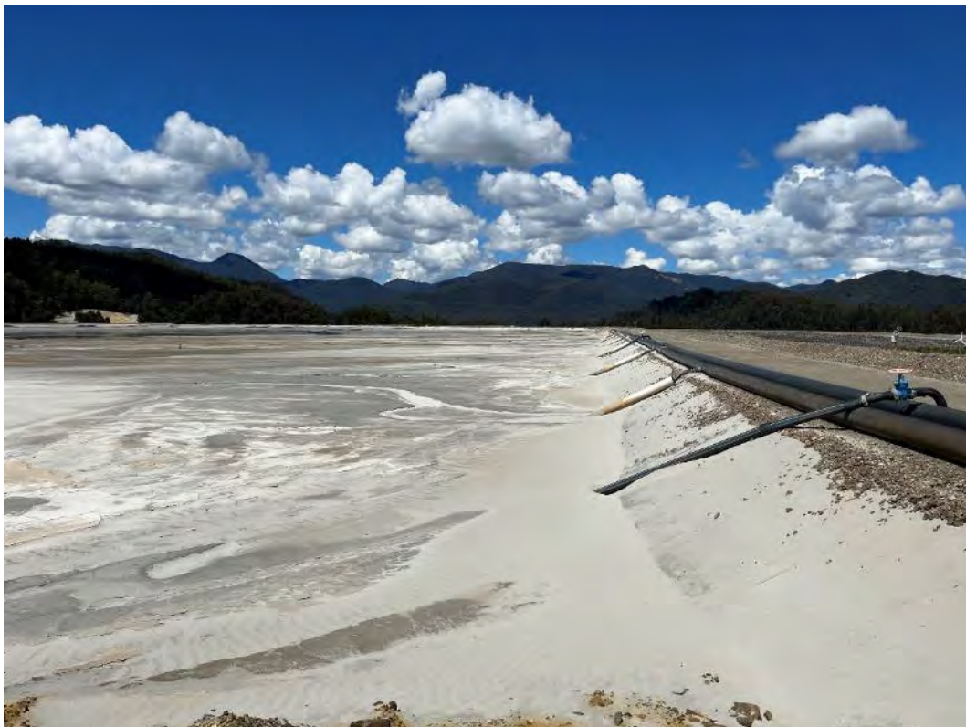
Photograph 32 – Tailings deposition from Stage 10, Levee Embankment, looking south west.
