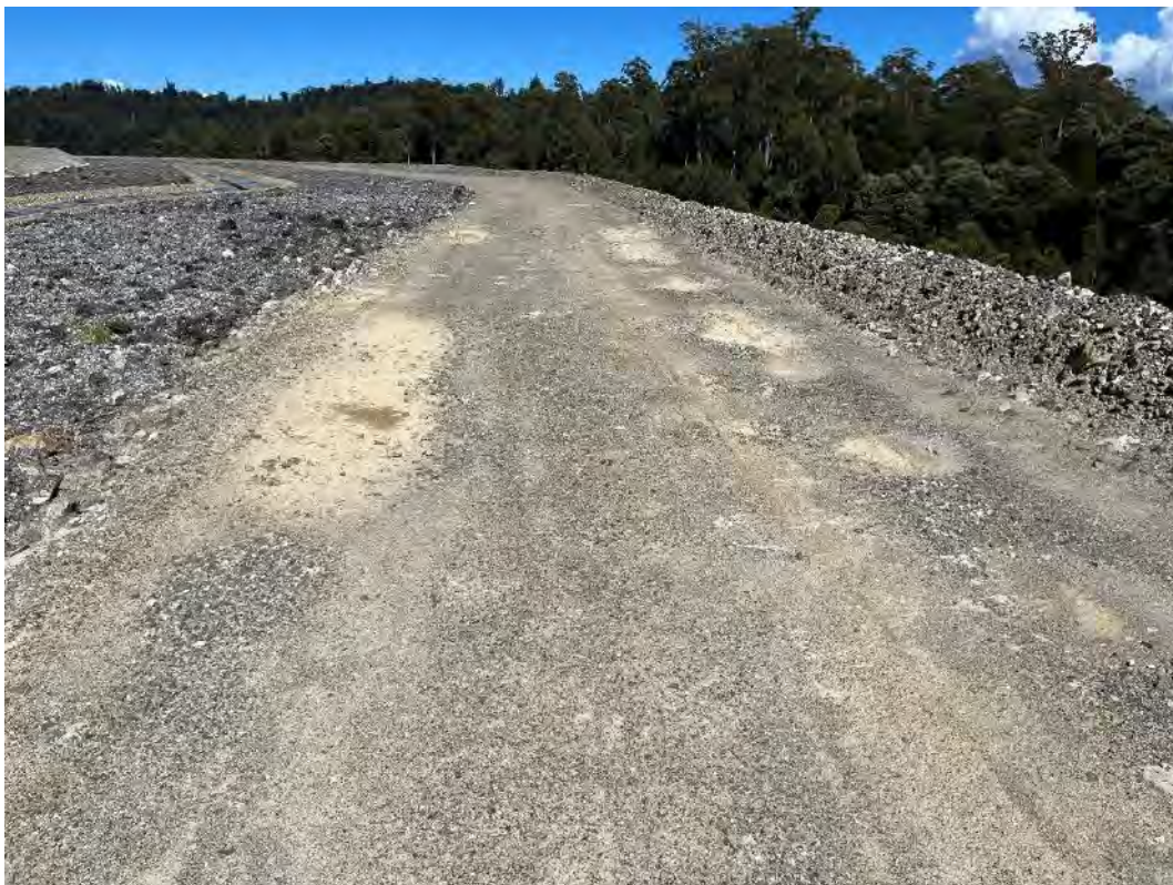
Photograph 28 – Levee embankment crest general condition.
