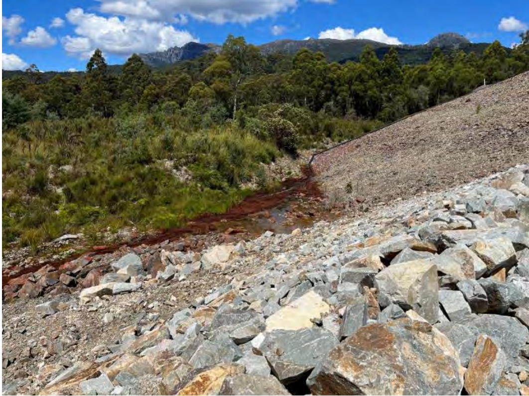
Photograph 11 – pooled seepage from original 5 Dam chimney drain outlet.
