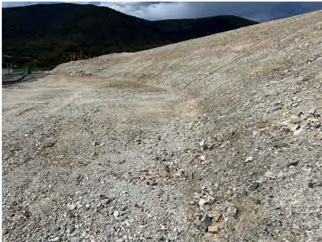
Photograph 35 – Overview of downstream face of screening bund, looking north.
