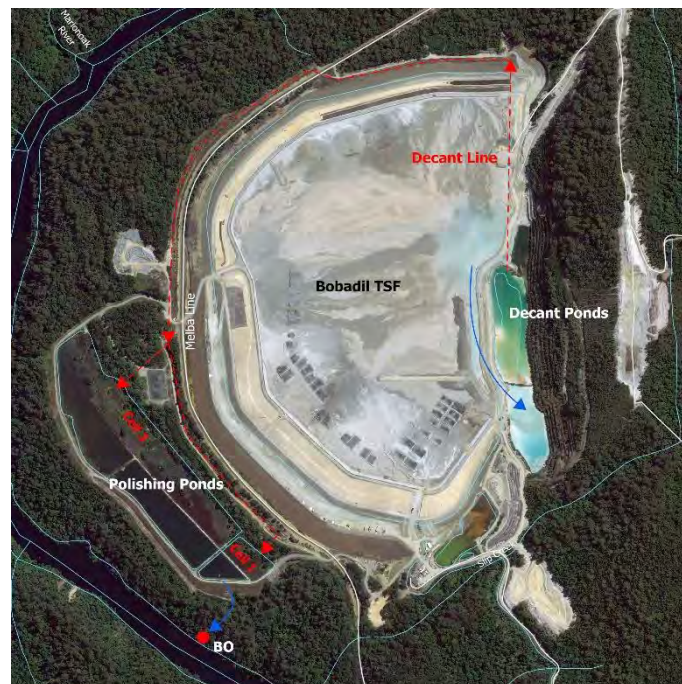
Figure 3-1. Bobadil TSF showing the main dam, Decant Ponds, decant line, Polishing Ponds, and the licenced discharge point from the Polishing Pond (BO).
