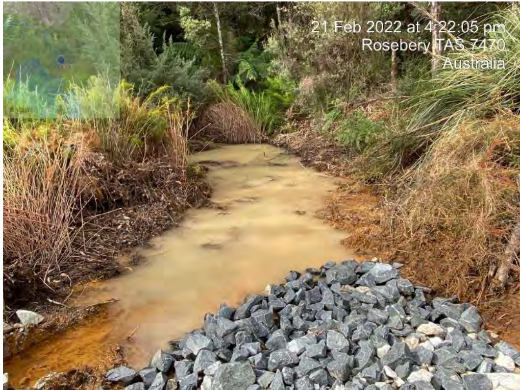
Photograph 19 – sediment laden seepage water (legacy seepage) downstream of the Stage 2 northern embankment buttress.
