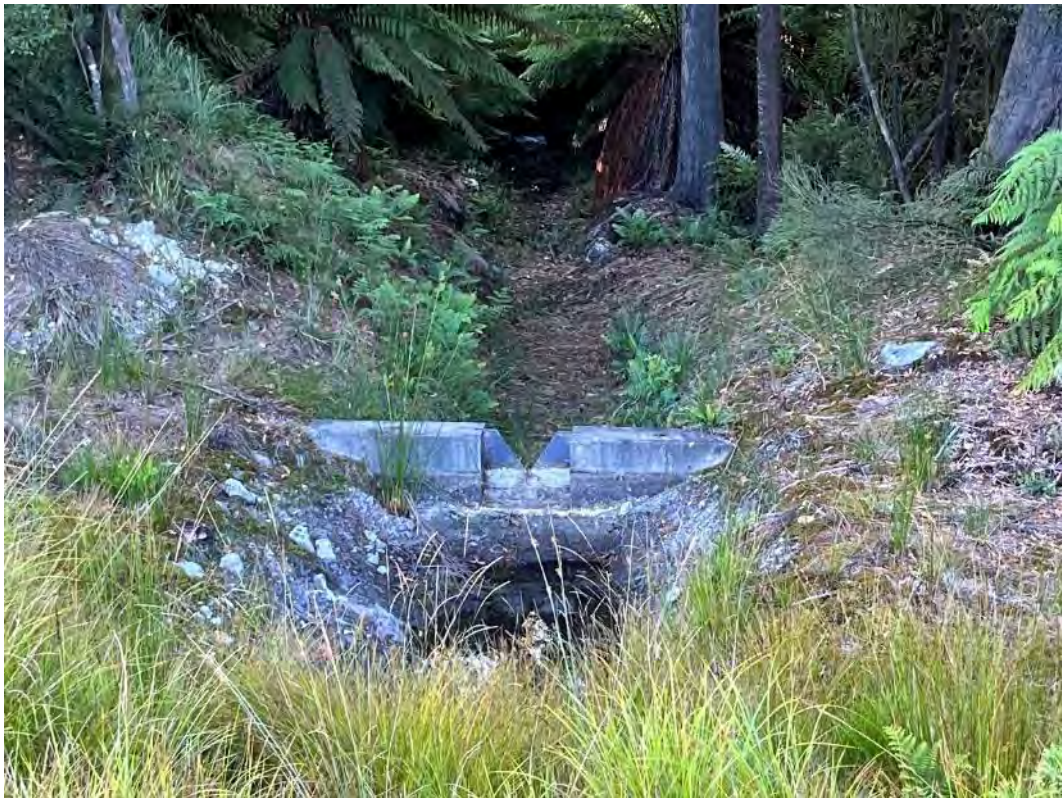
Photograph 42 – Polishing Pond –V-notch weir (VW 3)
