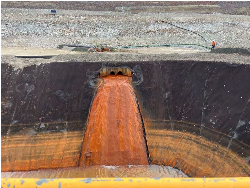
Photograph 14 – Culverts into the SCP from v-notch 4.
