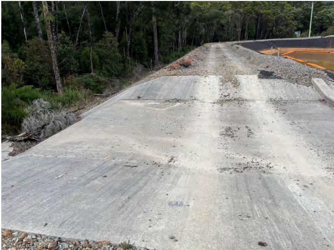
Photograph 15 – SCP spillway, clear of obstructions.
