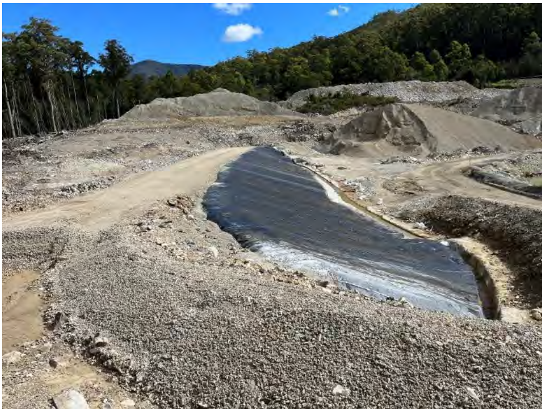
Photograph 24 – southern embankment, upstream face and liner.
