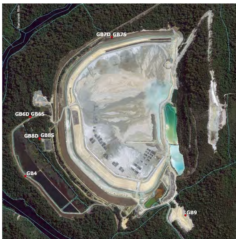
Figure 6-1. Location of groundwater monitoring bores near the Bobadil TSF.
