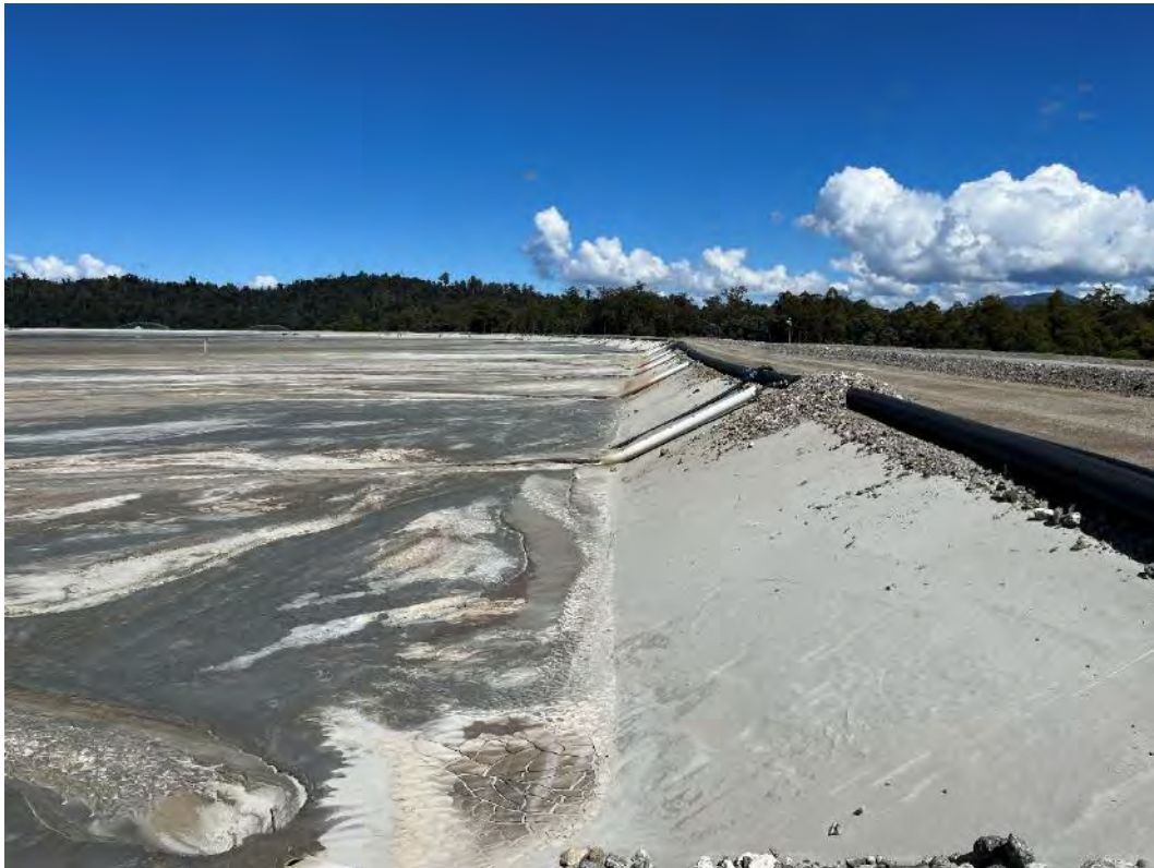
Photograph 11 – northern embankment crest (Stage 10), looking west.
