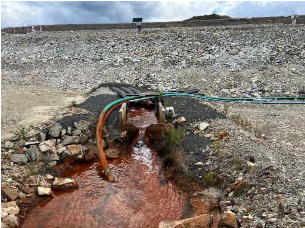
Photograph 13 – v-notch weir 4 downstream of the Stage 2 northern embankment buttress.
