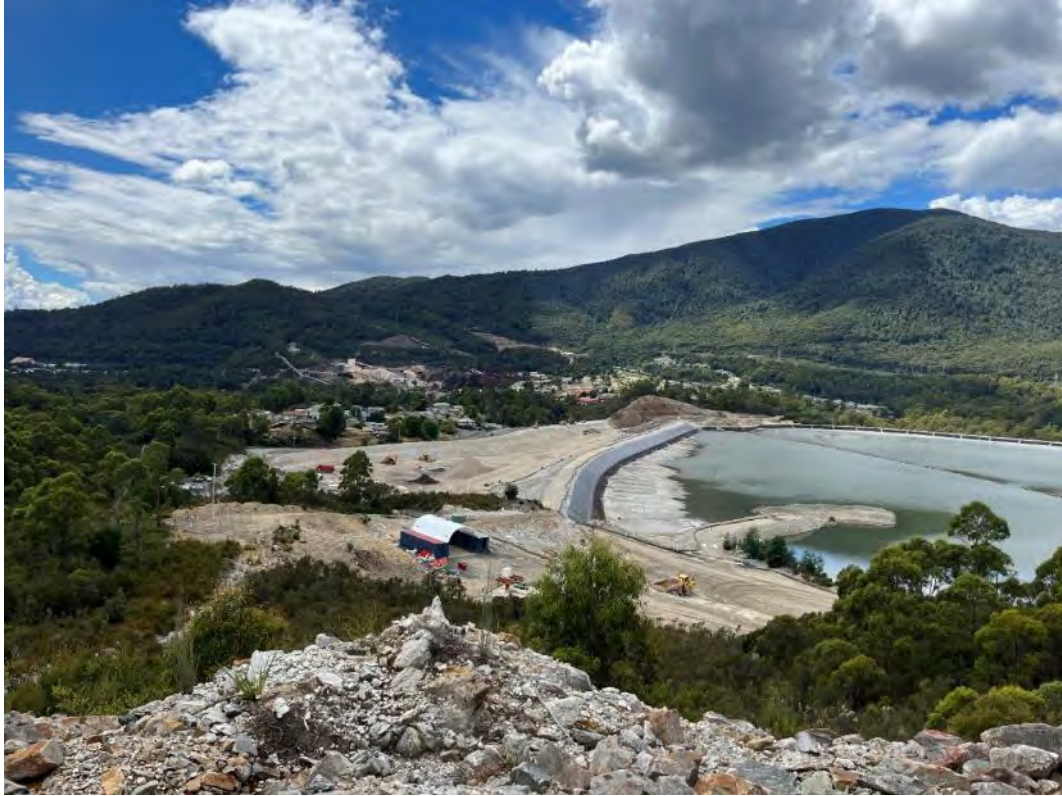
Photograph 29 – overview of western embankment, looking north from CWDD.
