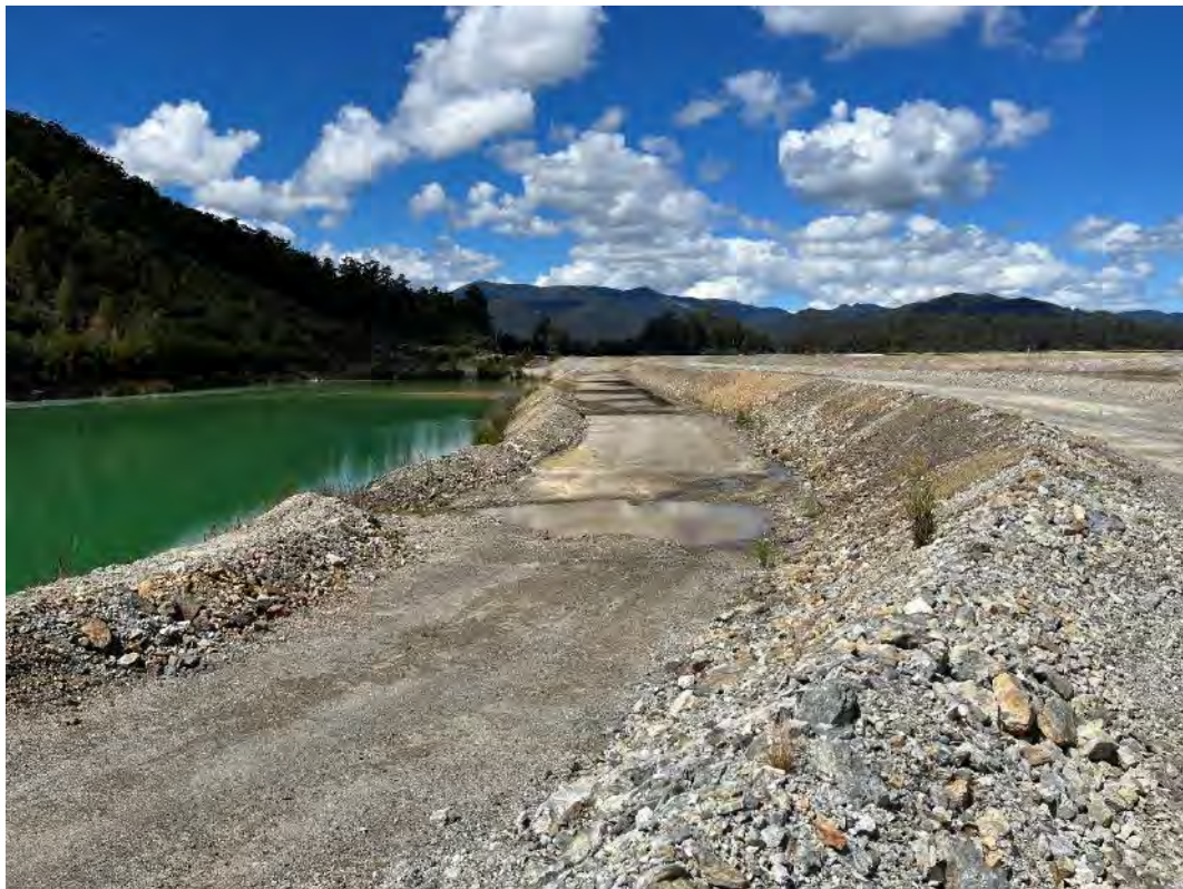
Photograph 26 – Decant filter wall crest, looking south.
