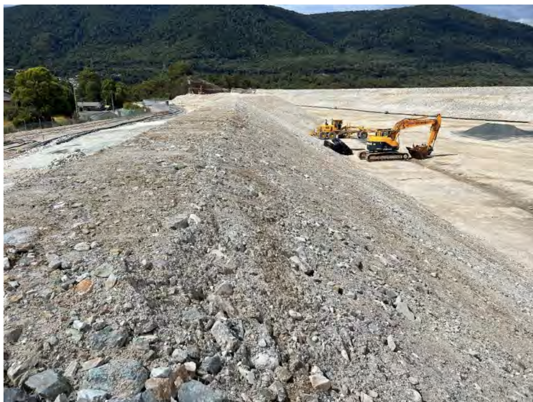
Photograph 36 – crest and upstream slope of screening bund.
