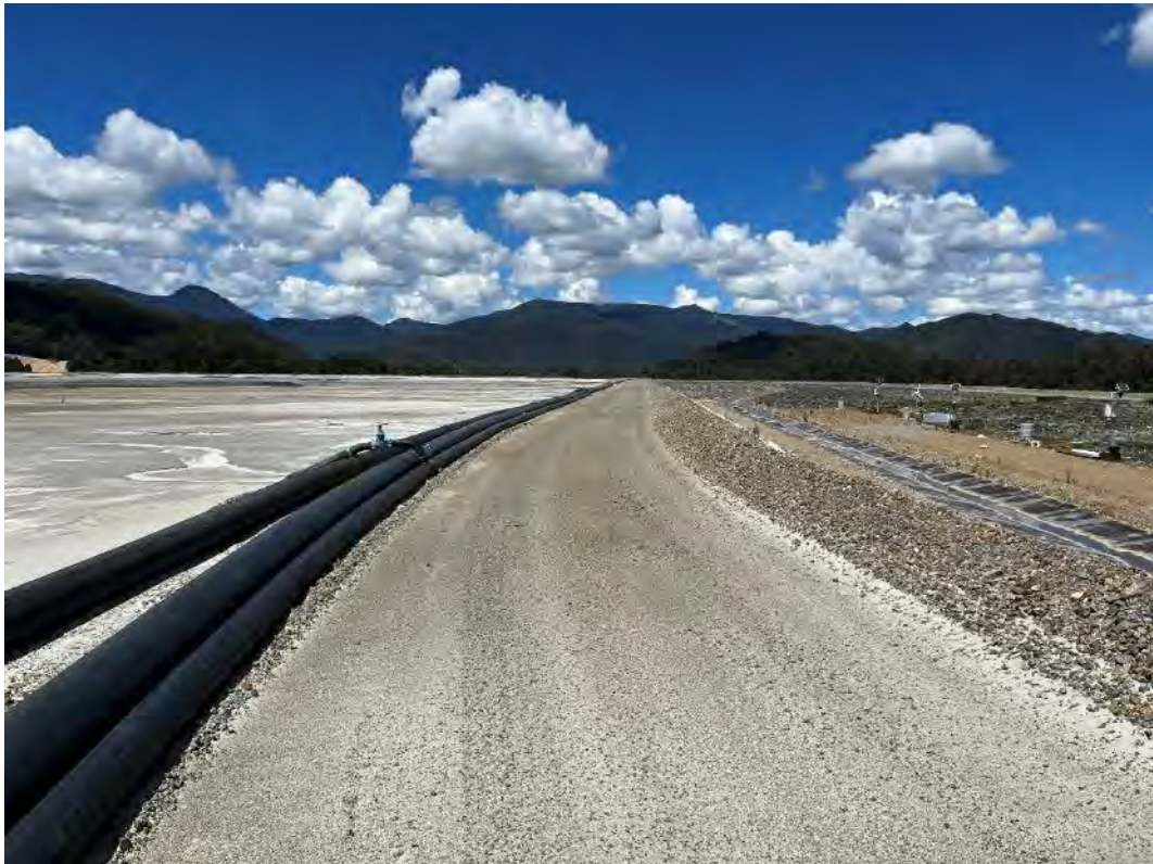
Photograph 23 – Levee embankment crest (Stage 10), looking south.
